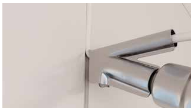
12a. Apply weldrod in the 3.5mm expansion gaps
