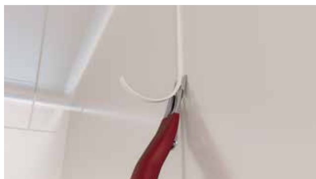
12.b After cooling, trim the weld rod with a Mozart blade
